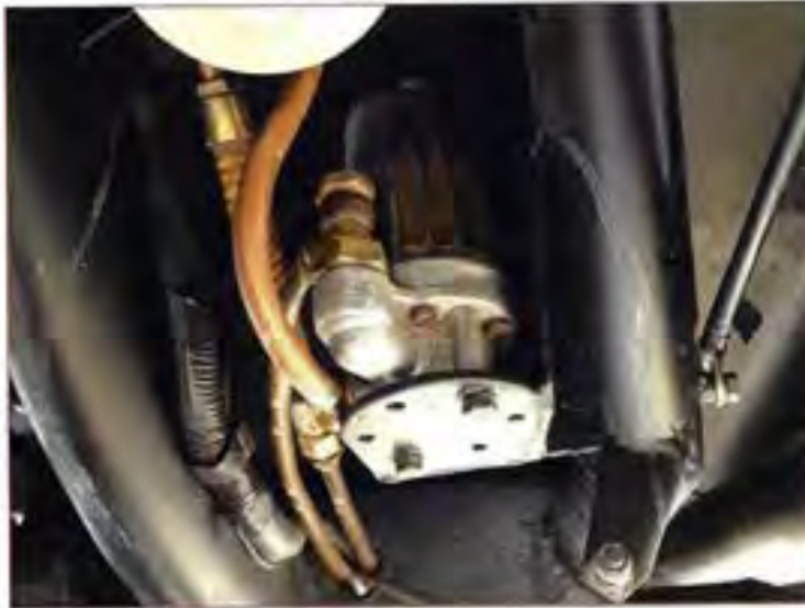
Pompa/o carburante Fuel pump/s
